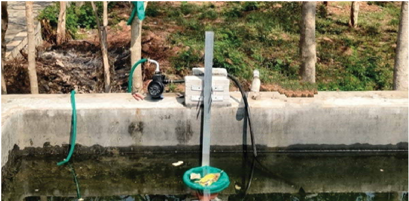
Figure 5. Final assembly and working of seabin model
