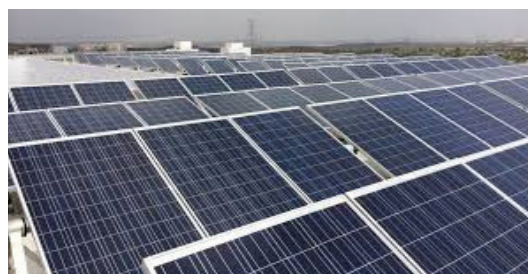
Figure 4. Solar panels on the building
