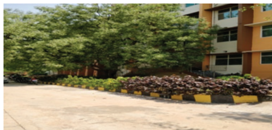
Figure 3. Landscape around the building
