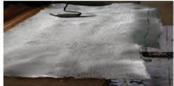
Fig-3 Removing the bubbles with a roller
