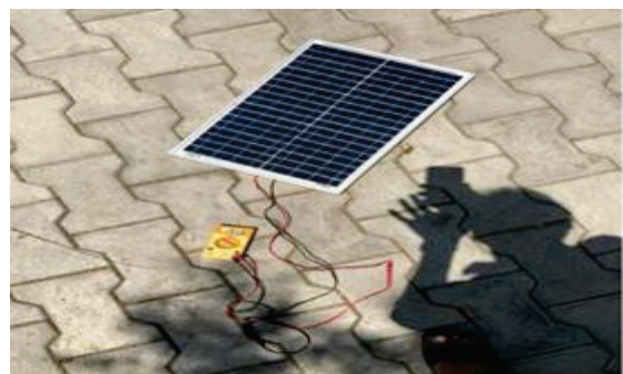
Figure 3. Open Circuit Voltage Measurement of a Solar Panel
