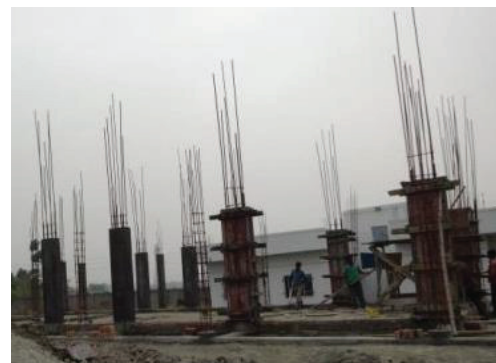
Figure 2. Traditional rebar extension for further lapping/splicing
