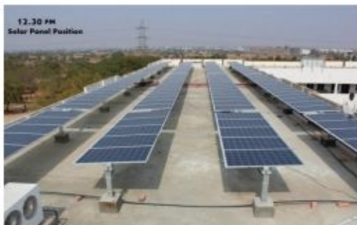
Figure 7. Single axis Tracking-Position of panels at 12:30 P.M
