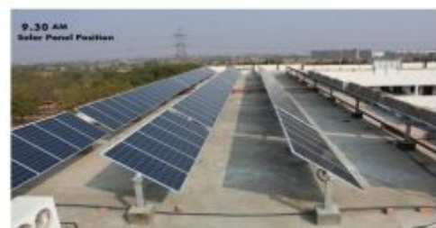
Figure 5. Single axis Tracking-Position of panels at 9:30 A.M
